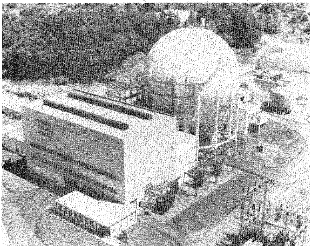
PICTURED ABOVE is the most recent view of the Yankee Atomic Electric Nuclear Powered Reactor. The reactor attained criticality on August 19, 1960. Low power testing continued until November 10. The turbine was rolled off Monday morning, January 16, and phased to the system about 10:00 P. M. that night. Generation was increased from 60,000 to 90,000, to 105,000 and then to 120,000 kilowatts at 3:25 P. M.
