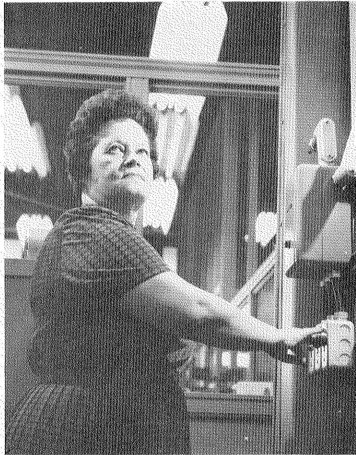
TAKEN FOR GRANTED — Louise Pettit, Receiving and Shipping Department, flips the light switch lighting up the X-720 area where she works. The electrical power involved here is just a "drop in the bucket". The annual Power bill to operate this plant exceeds $60,000,000.
