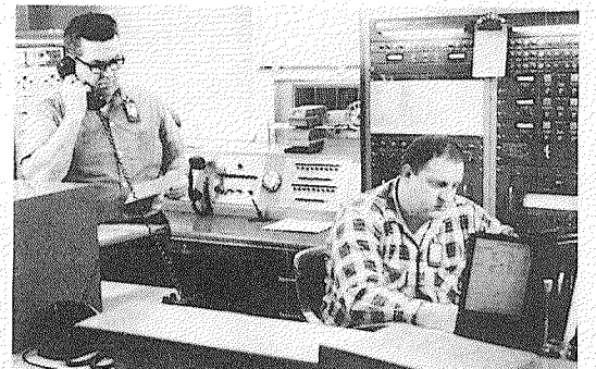
READY FOR AN EMERGENCY. Jim Foster (l) and Charles Osborne (D-113) man the fire and sprinkler monitoring system. In cases of emergency the monitoring system enables firemen to quickly pinpoint the troubled area. GAT has 350 automatic sprinkler systems, they contain over 150,000 sprinkling heads. Supplementing the sprinkler systems are 380 strategically located fire alarm boxes. By comparison the Portsmouth — New Boston area has a total of 275 fire alarm boxes.
