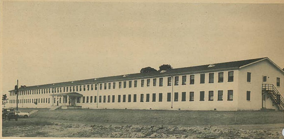
Living accommodations for approximately 300 jobsite workers were made available recently with the opening of Piketon Enterprise's new men's dormitory pictured above on state route No. 30 near the north boundary of the project. The two story structure, made of concrete block, is 325 feet long and has 100 rooms 12 by 16 feet. Owner-manager Jack Hatterick of Cincinnati said he also plans to build a restaurant adjacent to the dormitory in the near future.
