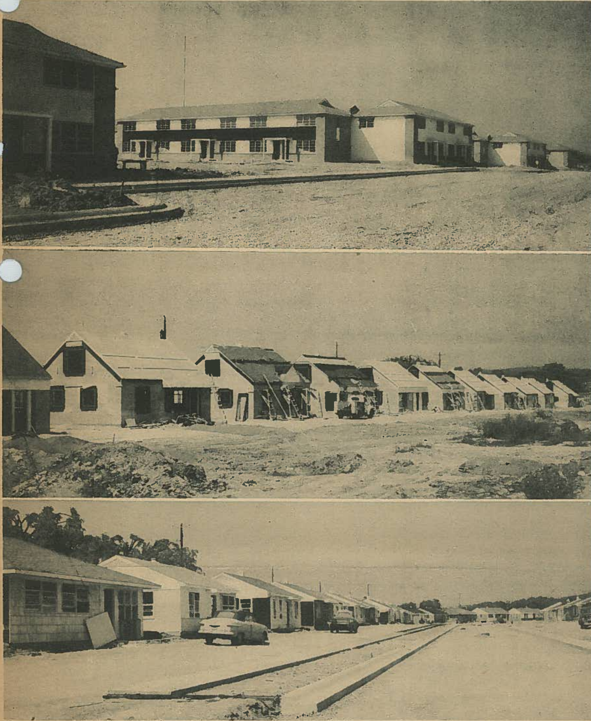
Three Federal Housing Administration projects nearing completion in the vicinity of the Portsmouth Area AEC project that will provide much needed living quarters for A-plant employees, are these shown above at Chillicothe and Waverly. The top photo was taken at Western Hills apartments in Chillicothe. Waverly Estates rental houses are pictured in the center photo and Waverly Heights sale units are shown in the lower picture. (See story on housing)
