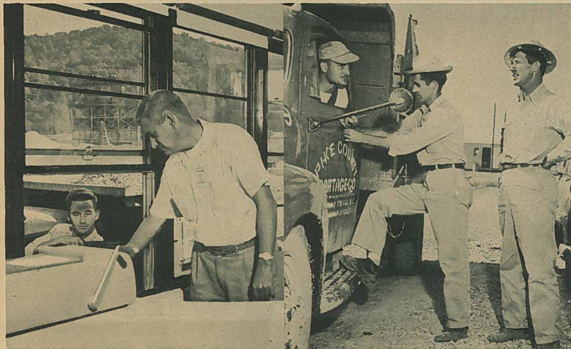
Over a million tons of rock have been taken from the quarry pictured above for use at the Portsmouth Area AEC project by the Ralph Rogers Company of Bloomington, Indiana. Pictured in the top right hand part of the photo are two of the four crushers in operation at the quarry located near Latham. In the lower left hand picture PKS Checker Walter Schauseil of Waverly is shown handing Driver Arizona Reno a scale ticket before heading for the jobsite. In the lower right photo Superintendent D. E. Wiginton, of the PKS Heavy Construction Division, watches Rock Dispatcher Carl Esham of Quincy, Ky., give a dispatch slip to Driver Bill Brandenburg at the jobsite.
