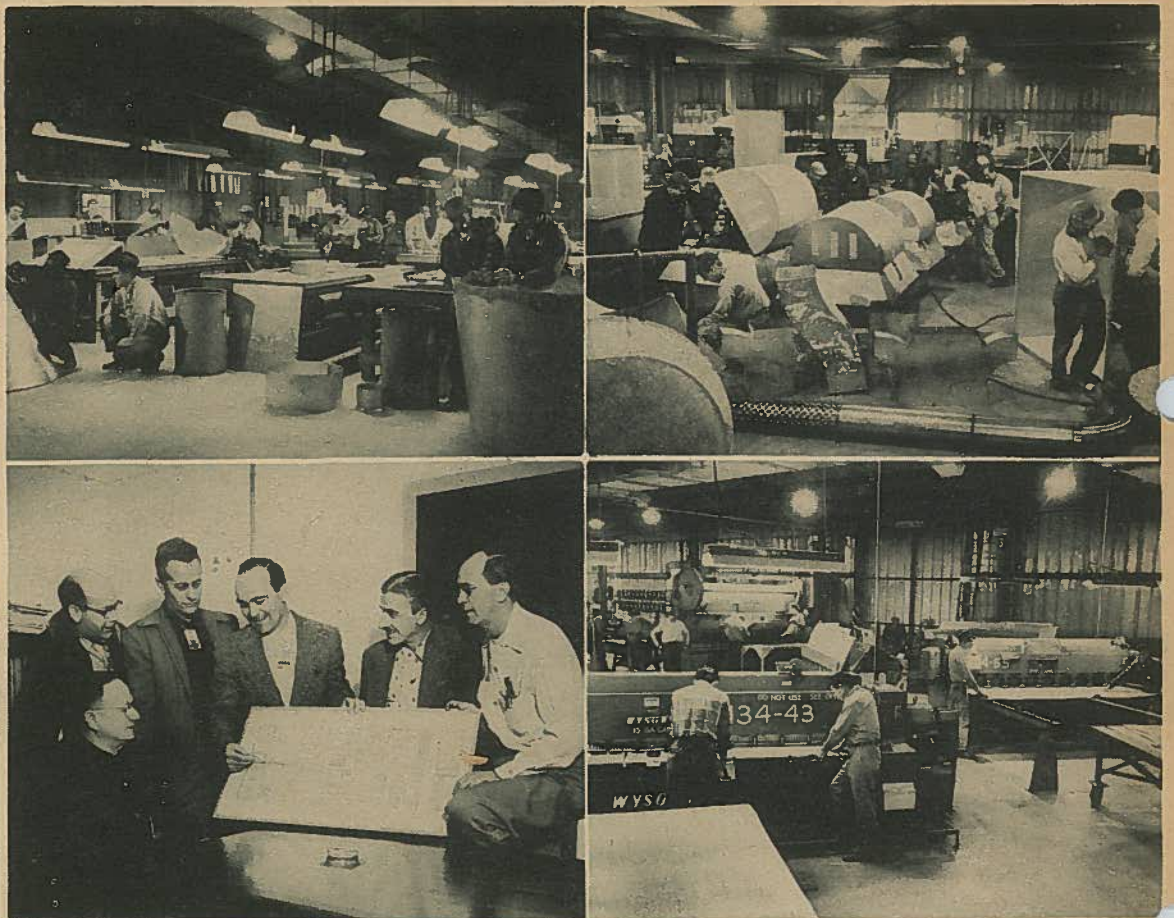
Pictured above are supervisory personnel and operations at the George Koch Sons, Inc., Field Sheet Metal Shop. Top left is the design and layout section. Top right, employees are shown in the assembly section, and lower right are pictured the big cutting and forming machines. In the lower left photo Assistant Division Superintendent Francis Walter points out a change in the make-up of the Sheet Metal Shop to General Superintendent of Sheet Metal Operations George Hoelscher (seated left), while looking on from left to right are: Assistant Division Superintendent Milo Shaw, Division Superintendent of Construction Ralph Simpkins, Shop Superintendent William Miller, and Assistant Shop Superintendent Joseph Baldwin.
