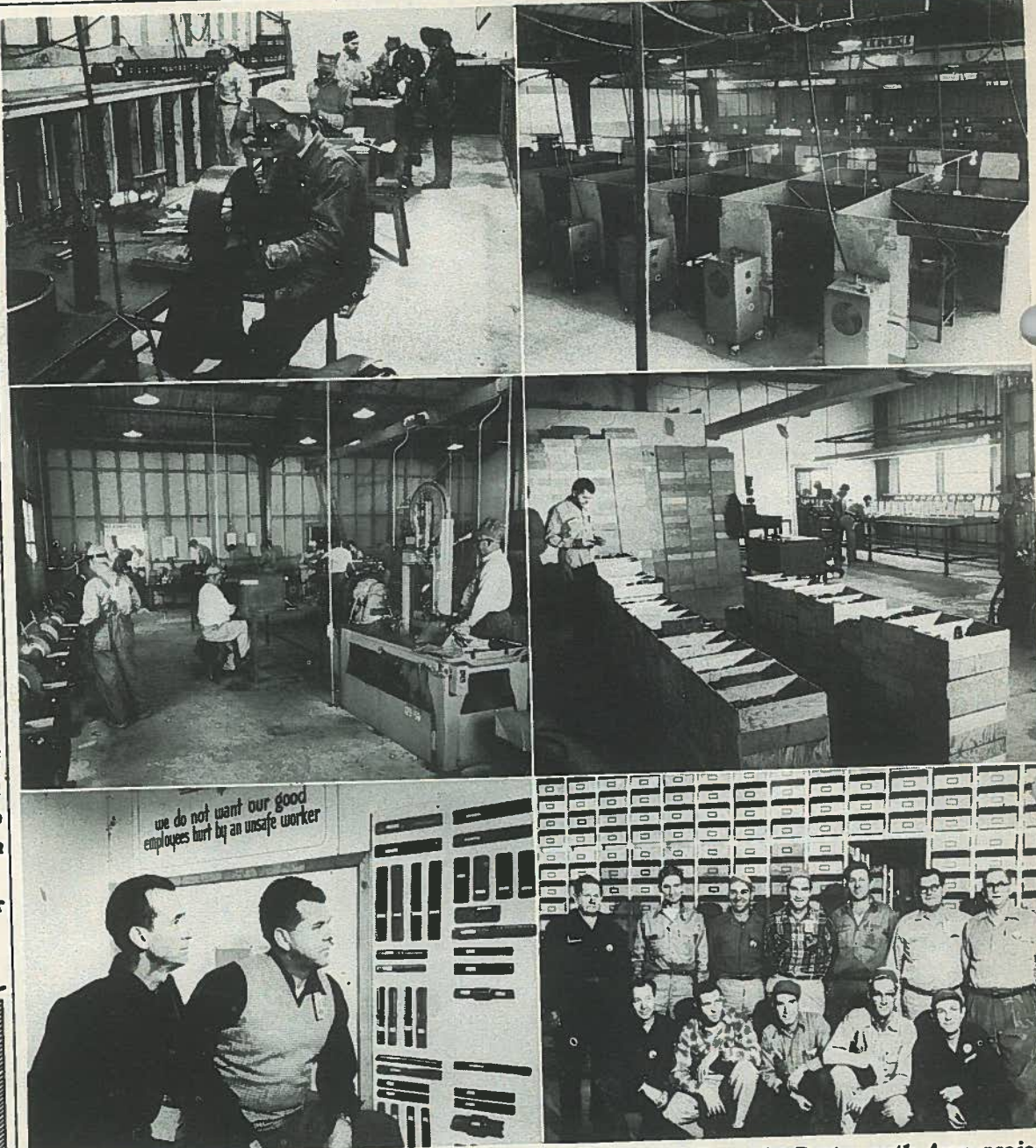
Pictured above in part is the story of the Grinnell Weld Test Lab on the Portsmouth Area project. In the upper left photo workers prepare material that will be used by welders being tested after applying for jobs. Upper right shows the individual booths that welders occupy while completing their tests. Center left is the machine shop where the welds are cut out, lathed, buffed, sawed or shaped. In the center right picture is the analysis room where each welder's work is thoroughly checked and rated, deciding whether or not he will pass. Lower left Weld Test Lab Superintendent D. A. Holder (left) and Assistant Superintendent W. T. Jackson look over board with specimens of proper and improper welds in the lab's reception room. Lower right are instructors and foremen who are a part of the Weld Test Lab's permanent personnel. Kneeling left to right are: Luke Lovett, A. R. Ferguson, H. E. Terry, T. R. Scott and Pete Adams. Standing left to right: Grant Rice, T. J. Bryant, M. L. Jones, A. E. Appleton, W. M. Green, W. H. Spronk, and T. H. Williams.
