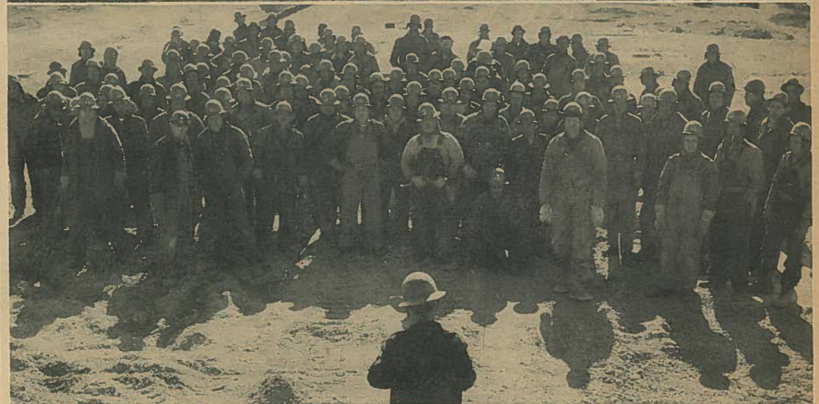
Pictured above are employees of the American Bridge Division of the United States Steel Corporation working on a structural steel fabrication and erection contract on the Portsmouth Area AEC project. In the top photo from left to right are: Timekeeper Warren Lorenzen, Assistant Superintendent Robert Anderson, Superintendent A. B. "Art" Drilling, Field Engineer W. O. Jayne, Assistant Timekeeper John Mullens and Safety Engineer W. W. Clasen. In the middle picture employees of the "yard crew" are shown at a weekly safety talk and in the lower photo workers of the erection group are pictured at a similar session being conducted by Safety Engineer Walt Clasen.
