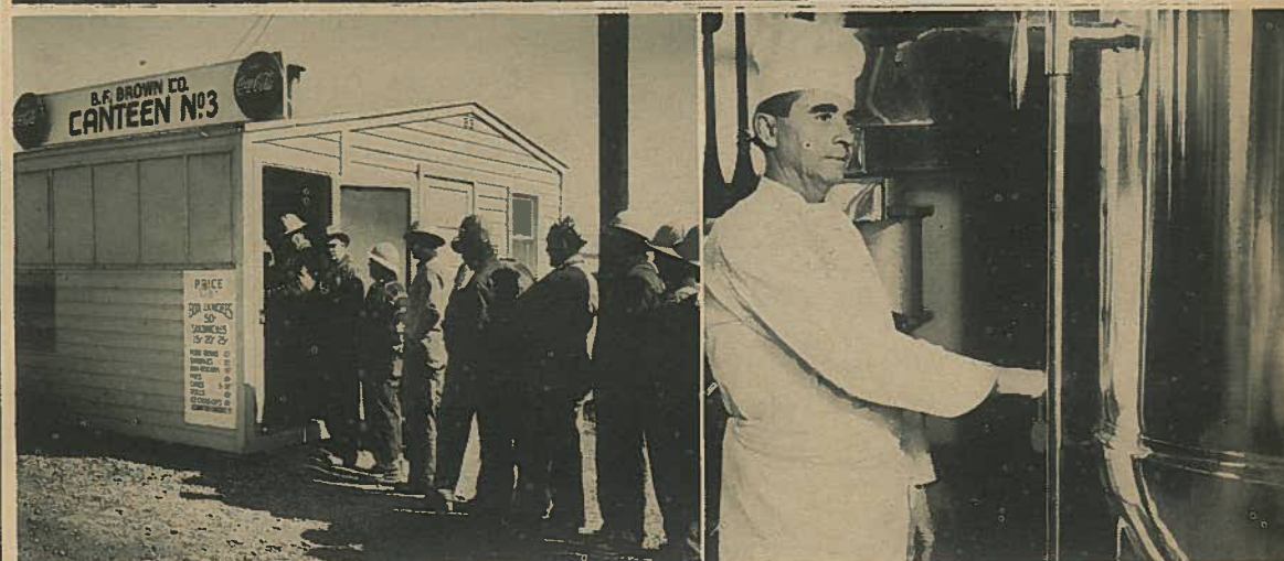
Shown above are several phases of the B. F. Brown Co., Inc. feeding program on the Portsmouth Area project. In the top photo an overall picture of the project cafeteria is shown during a typical lunch period. In the middle picture employees file through one of the four food lines in the cafeteria, and lower left "field" employees at the project line up at one of the ten field canteens operated by the B. F. Brown Company. At lower right Head Chef George Eakens checks on the cafeteria's 125-gallon coffee maker.
