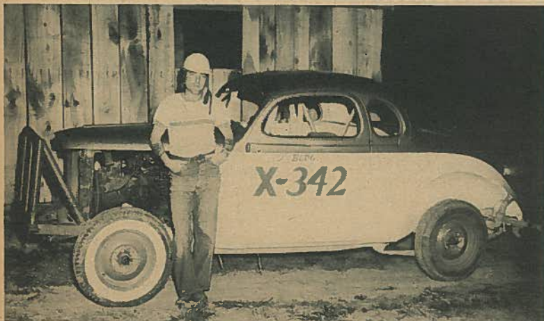
Standing beside his 1937 Plymouth "stock car" racer which he will enter in events at the Atomic Speedway is Phil Fitzsimmons, a Grinnell Corporation pipefitter on the Portsmouth Area project. Fitzsimmons' racer is numbered after the project building on which he is employed. (See story on page 3).
