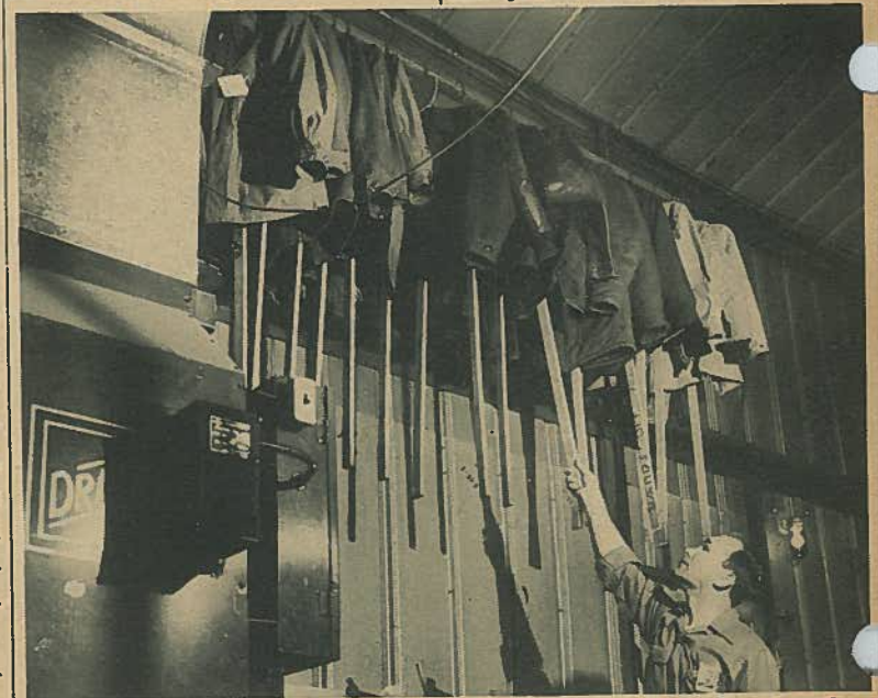
Six elevated coat racks, like the one pictured above showing Geo. Koch Sons, Inc., Assistant Division Superintendent Francis Walter hanging up his jacket, have been constructed in the Koch Field Sheet Metal Shop. Walter, who is in charge of the Field Sheet Metal Shop, said his idea for the racks was not entirely original but it presented a way to remove clothing from around machines and also gave more floor space. AEC Safety Chief W. C. Crozer said the racks were one of the most unique ideas he had ever seen and certainly showed good safety practices were being exercised. Coats are placed on a wooden-type hanger with a hook on top. The hangers are connected to a four and a half foot stick which enables the garments to be placed on the steel rod suspended approximately 12 feet off the floor.
