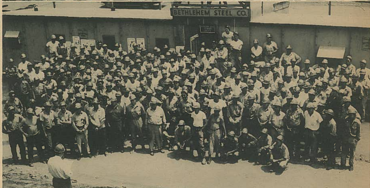
Pictured above are employees of the Bethlehem Steel Company's Pittsburgh Erection operation at the Portsmouth Area AEC project. In the top picture from left to right are: Field Clerk Lee Lawton, Field Supervisor Ted Wolfe, Field Supervisor Joe Morgan, Welding Superintendent D. M. Hood, General Superintendent J. B. Gibson, General Foreman John Kukoda, Field Engineer Jim Minnich, Office Manager Frank Zundt, Field Supervisor F. Kucharski, General Foreman Bill Shaw. Shown below are several hundred Bethlehem employees attending one of the weekly safety meetings being conducted by Superintendent J. B. "Jim" Gibson.
