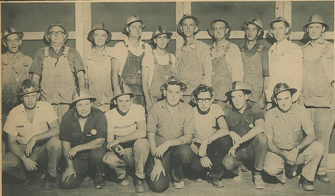
This Peter Kiewit Sons' Co. general Carpenter crew employed in the X-326 process building was selected to appear in this edition of THE ATOMIZER on the basis of its over-all job performance and safety record. Kneeling left to right are: General Foreman R. L. Smith, Carpenter Helpers C. Himes, J. C. Clemons, R. L. Bradshaw, D. W. Brown, K. H. Back and Foreman D. H. Beckley. Standing are: Carpenters M. J. Morgan, J. S. Pickett, M. H. Lemaster, H. C. Townley, L. M. Stone, A. A. Rohlfing, P. M. McFall, A. Prater, J. D. Ortkiese and T. R. Lee.
