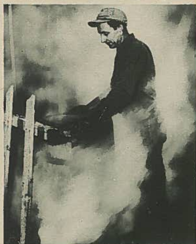
Laborer Ray Robinson holds a barrel over the steam nozzle as the high temperature steam swirls around him.
