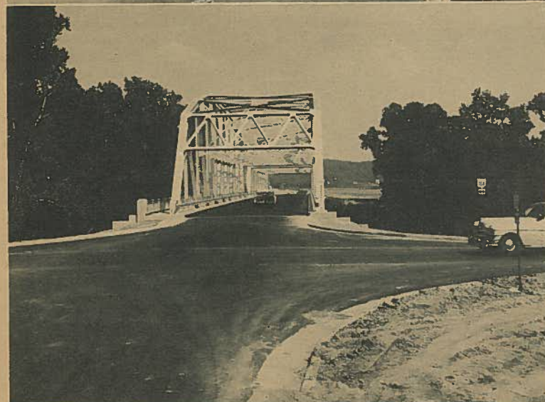
Another link was added to the chain of modern highways and bridges in the A-Plant area Friday afternoon, August 12, when the new strip of Route 124 and bridge spanning the Scioto River was opened to east-west traffic. By-passing Piketon completely, the highway joins the previously completed route near the State Highway Department Headquarters north of the project, and extends west across the Scioto River bridge; intersecting Route 104 south of Jasper and continuing through to old Route 124 east of Jasper. The top photo was taken from an overhead on Route 23, looking west toward the new bridge across the Scioto. The lower photo shows traffic travelling east on the new span at the intersection of Route 104 and the new highway south of Jasper.
